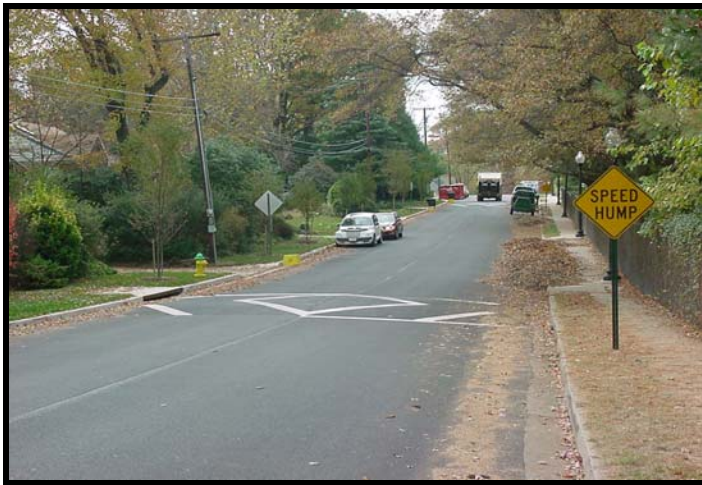
27 th Street North
